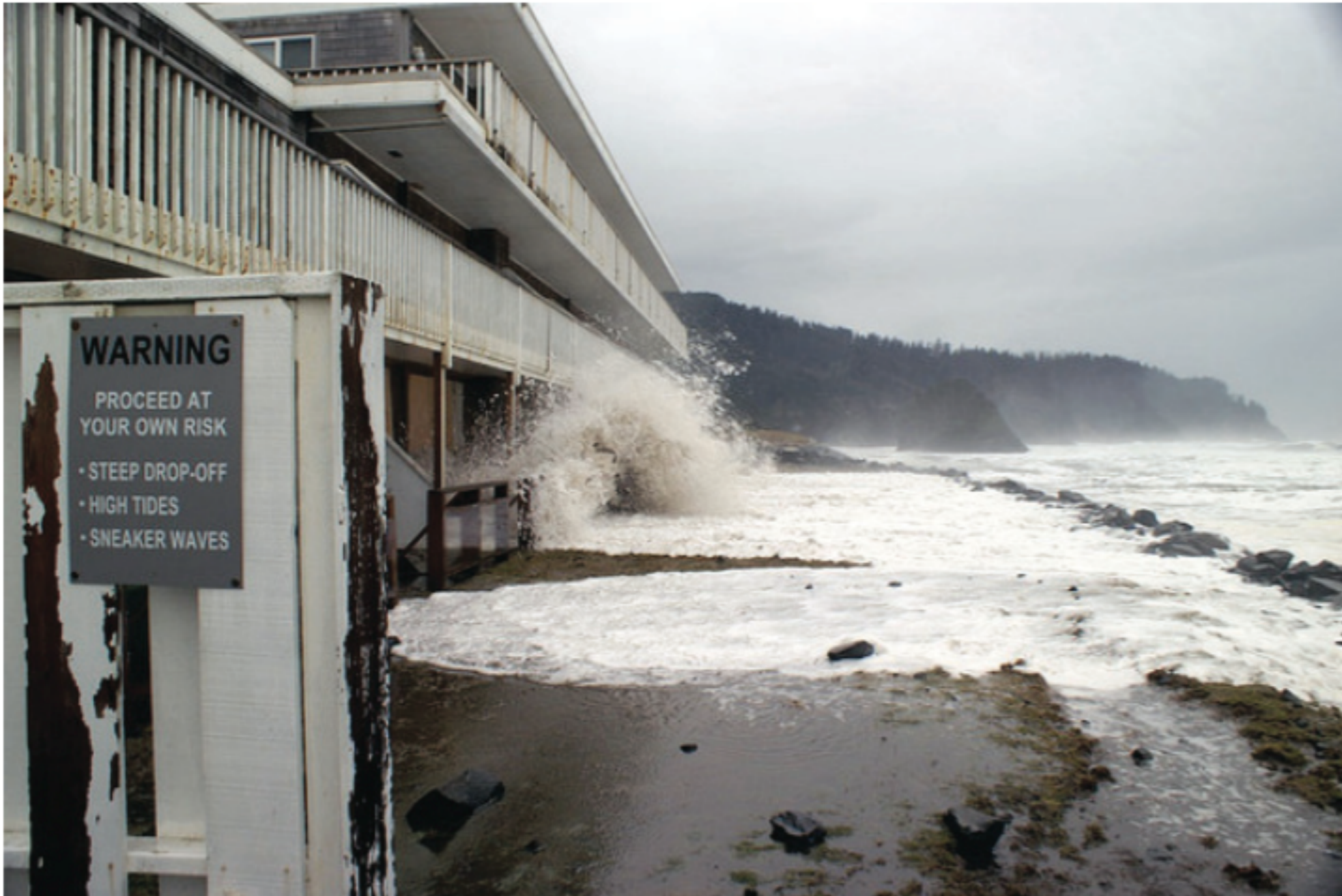
FIGURE 1.3 High surf during a high tide of nearly 2.7 m removed the front lawn of the Pacific Sands Resort at Neskowin, Oregon, on January 9, 2008. SOURCE: Courtesy of Armand Thibault.
